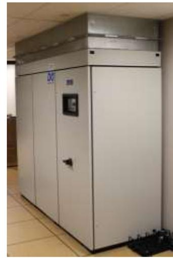
CRAC unit with plenum installed in the ceiling plenum for hot air intake
