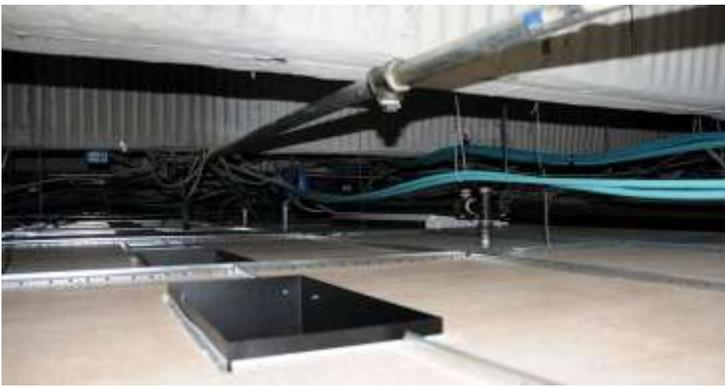
View of the ceiling plenum with cut-out and installed chimney.
