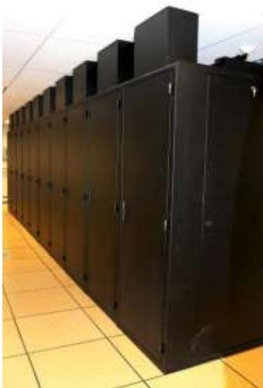
The concept behind the configuration proposed by Great Lakes, reduced the amount of "whitespace" (open area that does not have active equipment running and therefore, does not need cooling). By reducing the amount of whitespace being conditioned, less energy is used by the HVAC (heating ventilation and air-conditioning) system, resulting in higher efficiencies and greater capacity to cool equipment.
