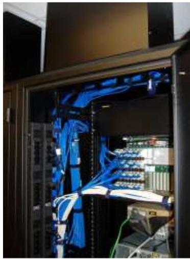
Cabling run from overhead to vertical patch installed toward the enclosure front which supports core switch
