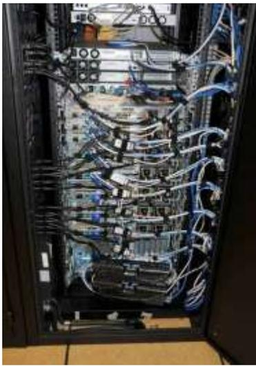
View of an enclosure using vertical patch and custom cable lengths
